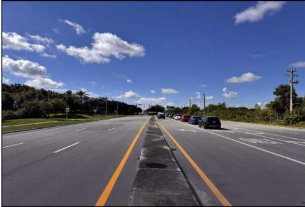
Looking south on Alternate A1A, subject is on the left
